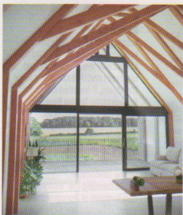
ABOVE At Black Barn, Douglas fir timbers taper upwards towards the large southern gable, creating a dramatic elevated roofline and framing magnificent views
